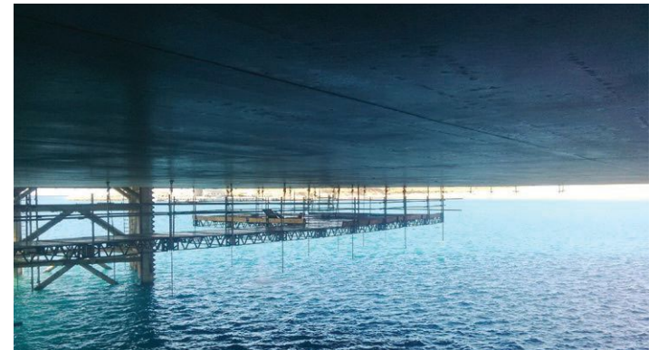
A patented and proprietary suspended access system, QuikDeck® provides factory-floor-like working conditions under areas where scaffold can't be built up from below.
