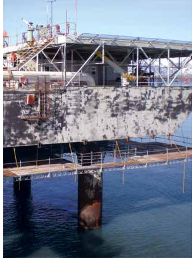
**Photo:** QuikDeck® in use for maintenance and repair of an offshore platform in Alaska.
