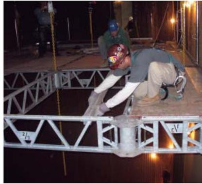
Safway electric hoists and modular staging systems fit through most boiler openings to help access areas for inspection, maintenance and repair. Use them in conjunction with Systems™ Scaffold.
