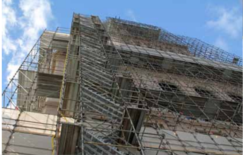
Safway's Systems Scaffold with lightweight aluminum decking and containment systems for increased safety encompassed the Travelers Tower.
